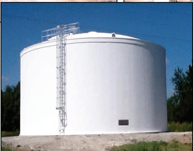
In our newsletter last quarter, we told you we had started construction on a new 1 million gallon ground storage water tank in April. This new water tank will help accommodate future growth to the city while helping to consistently serve Mayfield with clean water and adequate pressure during times of scheduled maintenance on our other water tanks.
